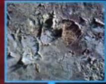
Intermittent heating is causing expansion and contraction of the synthetic coating and subsequent loss to the paint layer
